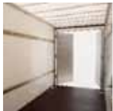
Roof, door & rails
